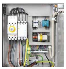
All electronic components installed in watertight cabinet
